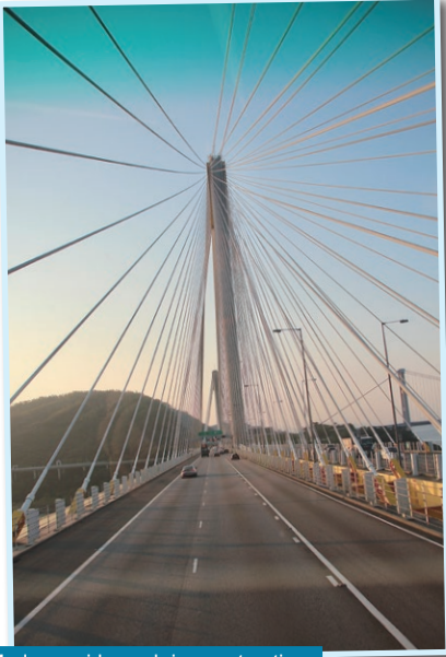
Modern spider web in construction.
